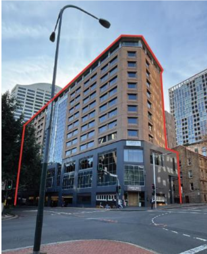
Figure 4 150 Day Street, looking north at Day and Bathurst Street Frontages (source: Planning proposal)
