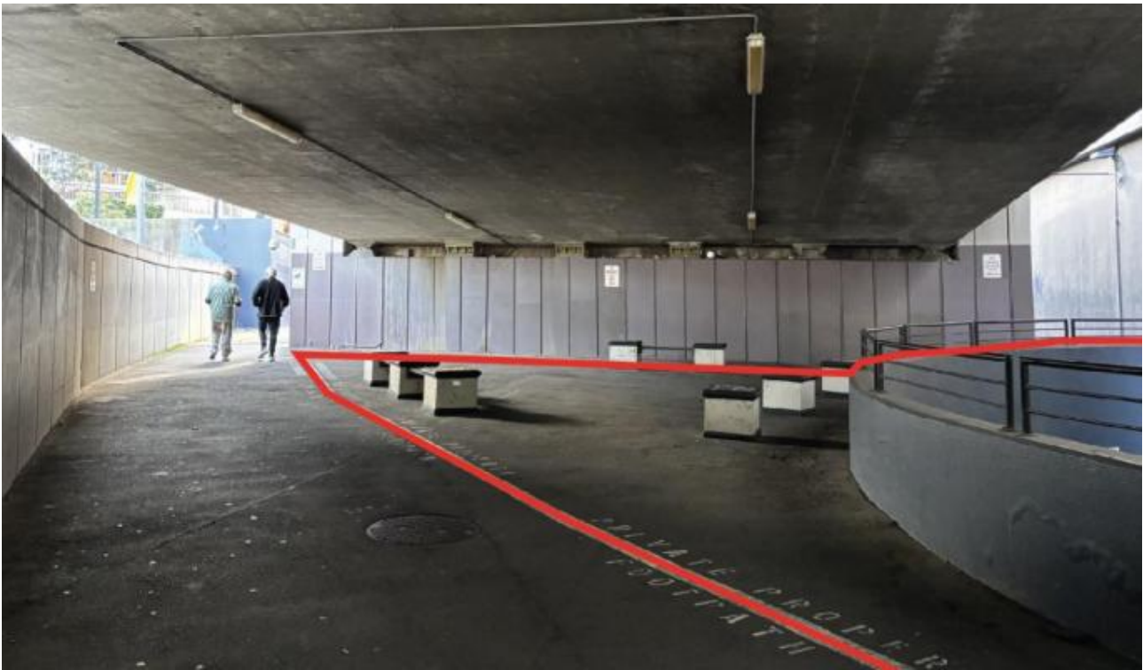
Figure 6 Pedestrian route underneath Western Distributor – site boundary in red (source: Planning Proposal)
